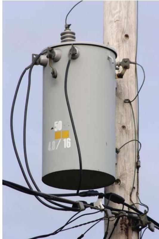
Figure 1. Power transformers are often used in power distribution lines.
