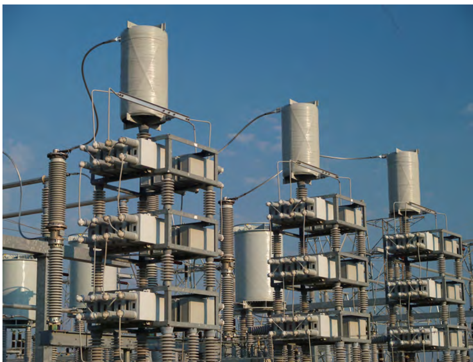
Figure 31. Bank of shunt capacitors used to compensate the voltage at the receiver end of a high-voltage ac transmission line.
