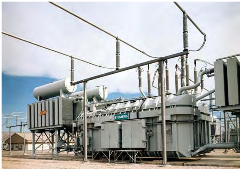
Figure 55. Phase-shifting transformer used to control active power flow through an ac transmission line in an interconnected power network (©Siemens AG 2014, all rights reserved).
