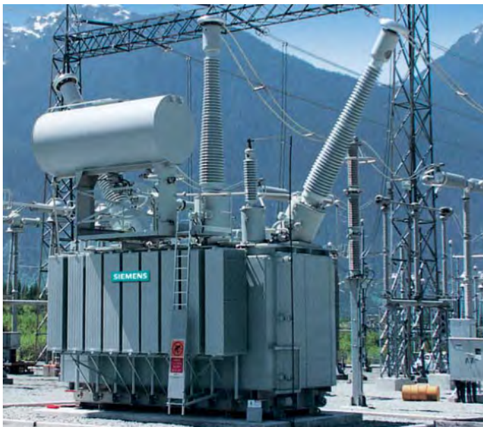
Figure 30. Shunt inductor (three-phase unit) used for voltage compensation of a high-voltage ac transmission line. Each long arm on the top of the unit shown in the picture is an insulator providing access to one end of an inductor (©Siemens AG 2014, all rights reserved).
