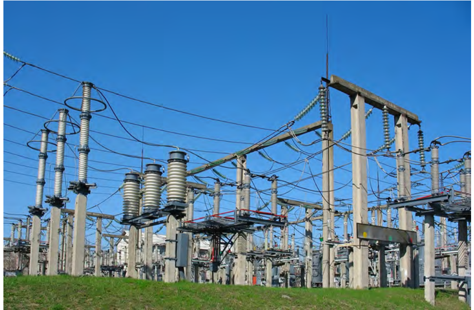
Figure 2. Transmission substation used for lowering the high voltage present in the ac transmission lines before the power is distributed to consumers.
