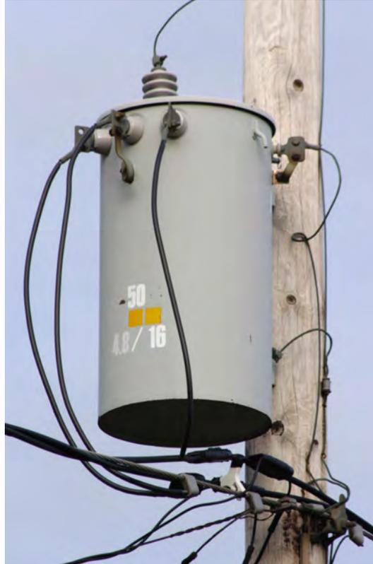
**Figure 1. Power transformers are often used in power distribution lines.<sup>1</sup>**
